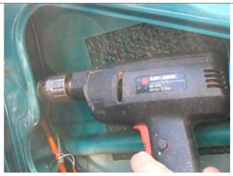
Access to inside is good so simply drill through the double skin from the inside using progressively larger drills. I started with 1/8" to minimise drill wander then a couple of others to the right size for the bolts.
