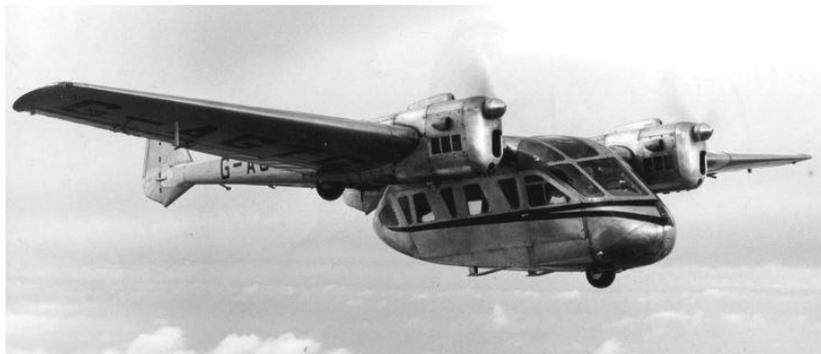
It was a twin-engine twin boom high wing monoplane using the Blackburn Cirrus Major engine of 155hp driving Rotol twin bladed variable pitch propellers. The passenger cabin could accommodate 5 passengers and the under-slung design meant that access was as easy as getting into a car. It was meant to have a range of uses with the publicity brochure showing scenes of a private / light executive transport or flying office, aerial pick up or even a float-plane or ski plane version.
